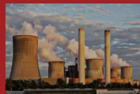
Coal & Thermal Power
